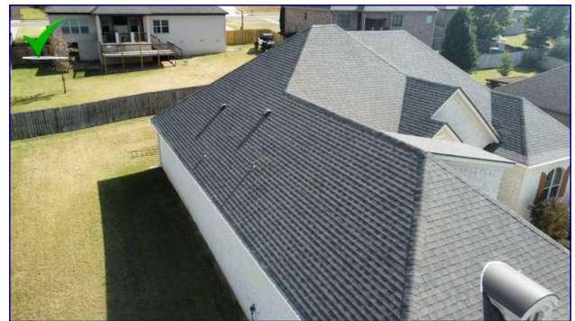
The Roof View
