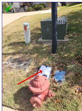
Main water shutoff location
