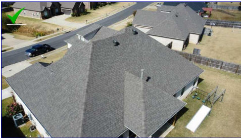
The Roof View
