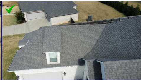
The Roof View
