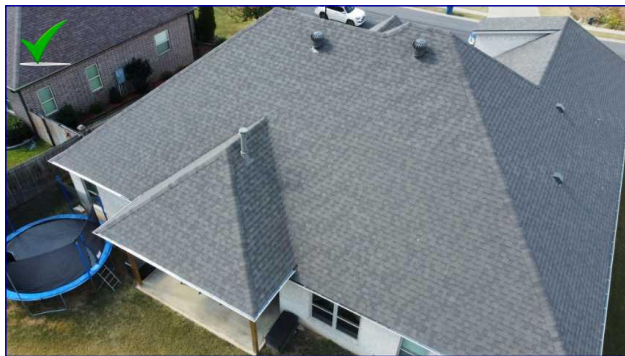
The Roof View
