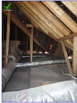
The Attic View
