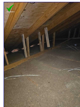
The Attic View
