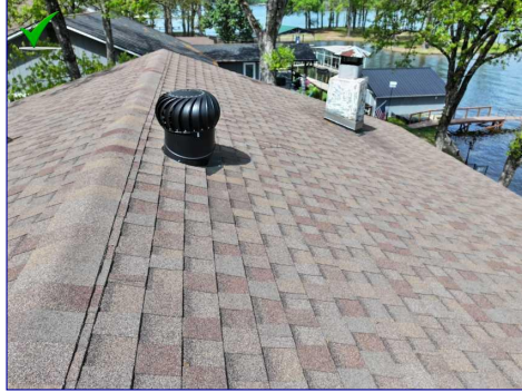
The Roof View
