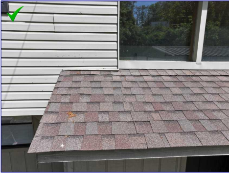
The Roof View
