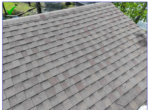
The Roof View
