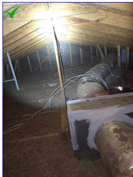
The Attic View
