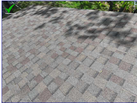
The Roof View
