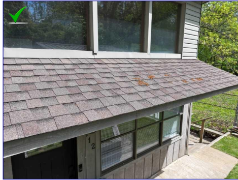
The Roof View
