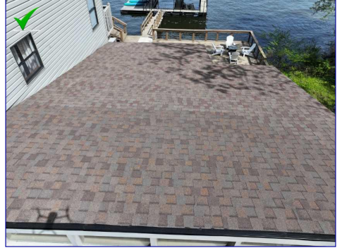
The Roof View
