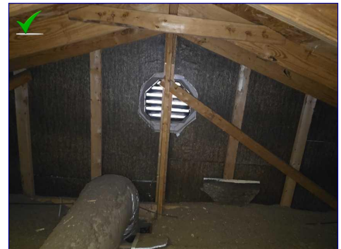
The Attic View
