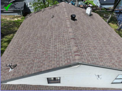
The Roof View
