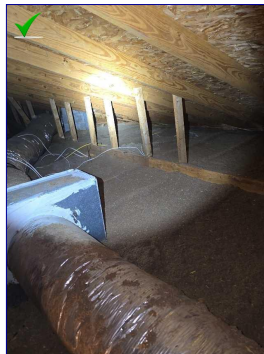
The Attic View
