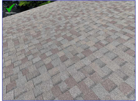
The Roof View
