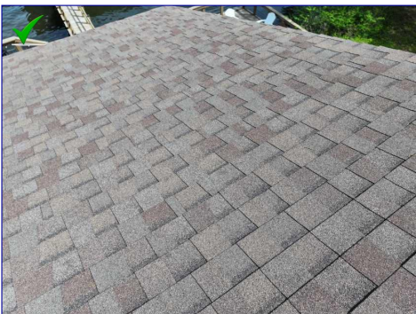
The Roof View
