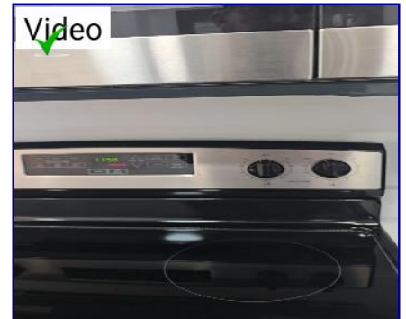
Exhaust fan and light operating
