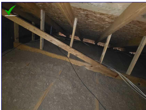
The Attic View
